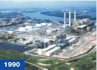
1990 Bang Pakong Power Plant (Kingdom of Thailand)
