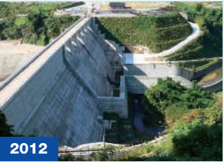
2012 Tatsumi Dam (Ishikawa Prefecture)
