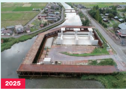
2025 Fukushimaagata Floodgate Main Structure (Niigata Prefecture)
