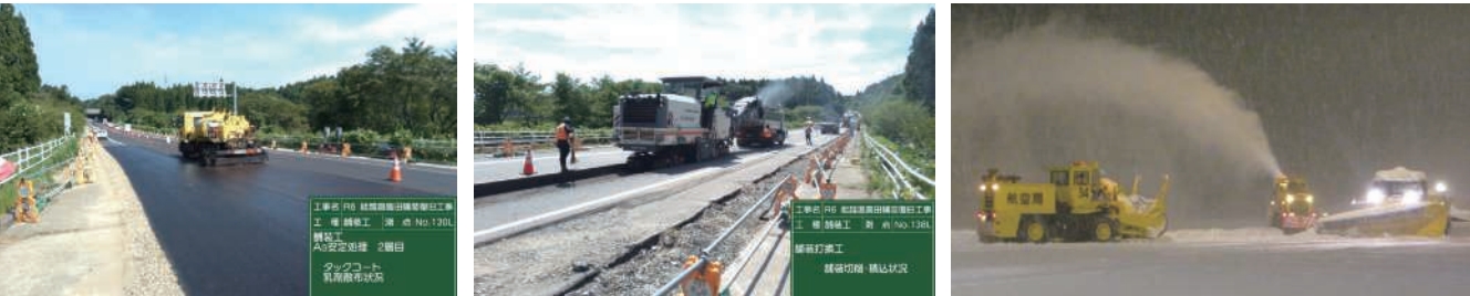
Status of Restoration Work in Noto
