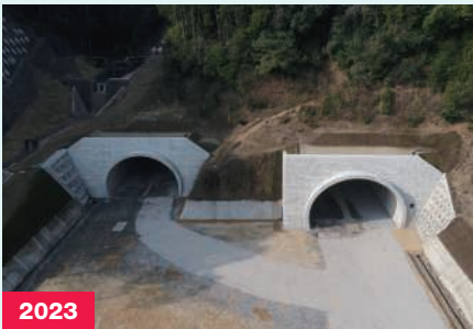
2023 Tokai-Kanjo Gifu Yamagata No. 1 Tunnel (Gifu Prefecture)
