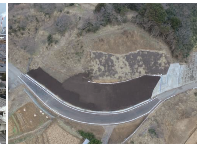
Road improvement works for disaster prevention, safety, and snow hazard mitigation on Primary Municipal Road 26 (proxy execution by the prefecture for remote island municipalities) (Niigata Prefecture)
