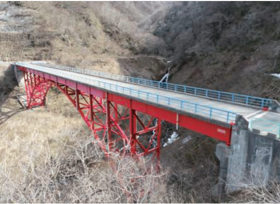
Kozuradani-Sasame Road Reconstruction and Disaster Prevention Project (bridge repair) by Niigata Regional Promotion Bureau Re-coating works (Gosen, Niigata Prefecture)
