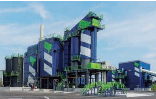
Panoramic view of Teraji Plant
