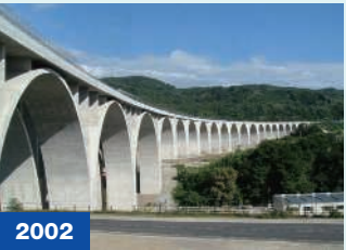
2002 Ueda Roman Bridge (Nagano Prefecture)
