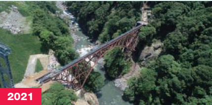
2021 Daiichi Shirakawa Bridge Restoration (Kumamoto Prefecture)
