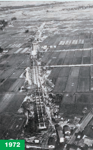
1972 Joetsu Shinkansen Kokonokamachi Viaduct (Section 2) construction
