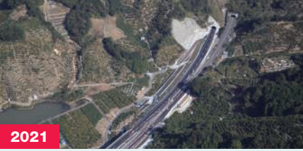
2021 Yanase Tunnel (Wakayama Prefecture)
