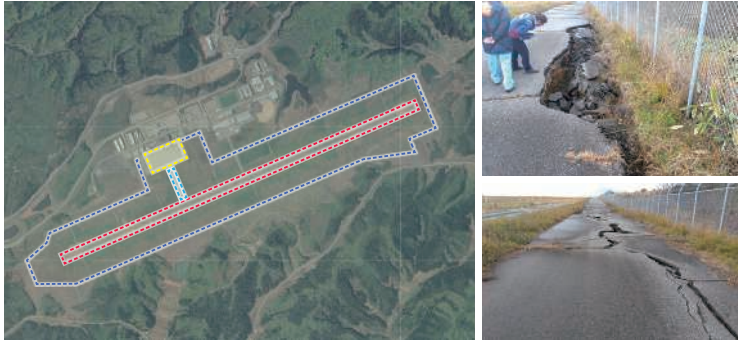
Noto Airport Damage Sustained at Noto Airport
