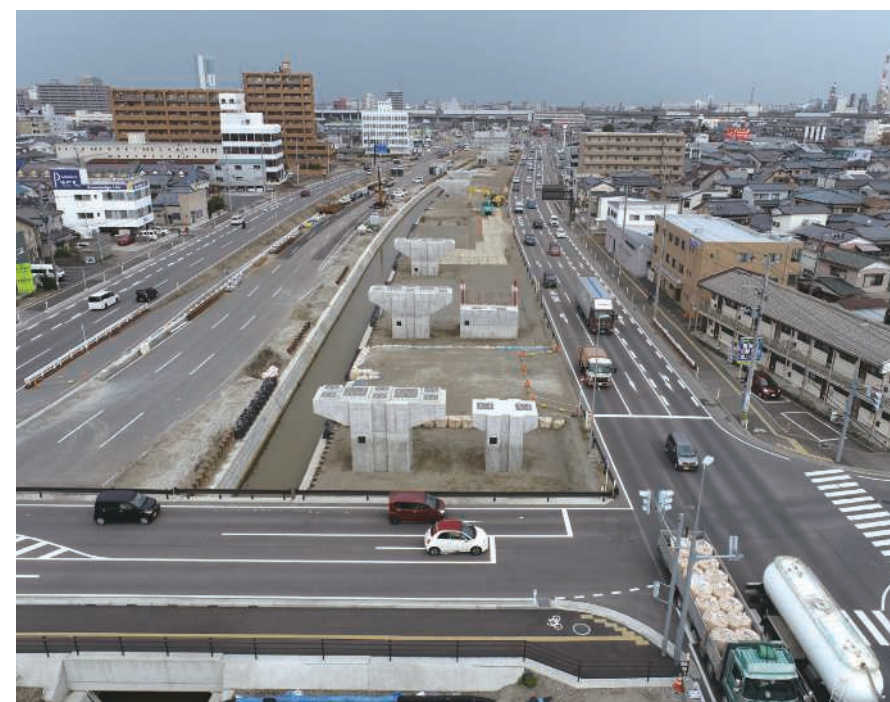
Construction of the substructures of the Kurinoki elevated bridge on the Kurinoki Road (Northbound P18-20, ONA2-P2) (Niigata Prefecture)
