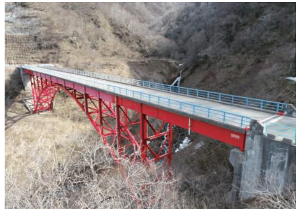
Kozuradani-Sasame Road Reconstruction and Disaster Prevention Project (bridge repair) by Niigata Regional Promotion Bureau Re-coating works (Gosen, Niigata Prefecture)
