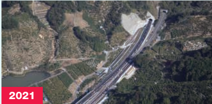
2021 Yanase Tunnel (Wakayama Prefecture)
