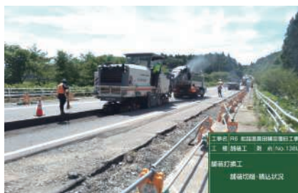
Status of Restoration Work in Noto
