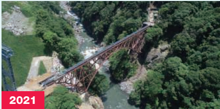
2021 Daiichi Shirakawa Bridge Restoration (Kumamoto Prefecture)
