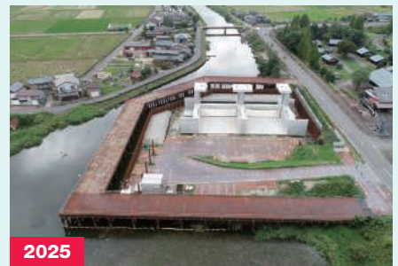
2025 Fukushimaagata Floodgate Main Structure (Niigata Prefecture)
