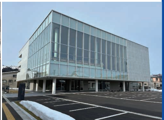
Uonuma City Lifelong Learning Center Construction Work (Niigata Prefecture)
