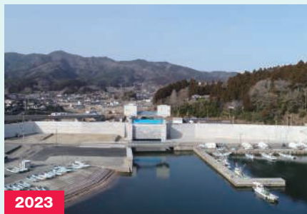
2023 Post-disaster reconstruction of Ryori Fishing Port and the coast (Iwate Prefecture)
