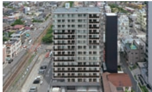
ANABUKI KOSAN INC. Tentative name: Alpha States Sumiyoshi II Construction Project (Nagasaki Prefecture)
