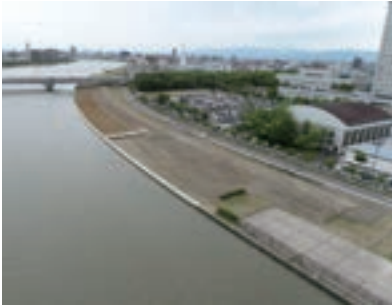
Ministry of Land, Infrastructure, Transport and Tourism Hokuriku Regional Development Bureau Shinanogawa River Downstream East Niigata District River Channel Excavating and Shinko-cho Yasuragi Embankment Exterior Construction Project Part 9 (Niigata Prefecture)
