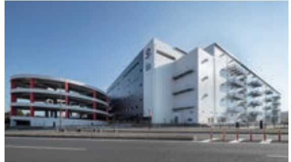
Urawa-misono Specified Purpose Company Tentative name: DPL Urawa-misono Construction Project (Saitama Prefecture)
