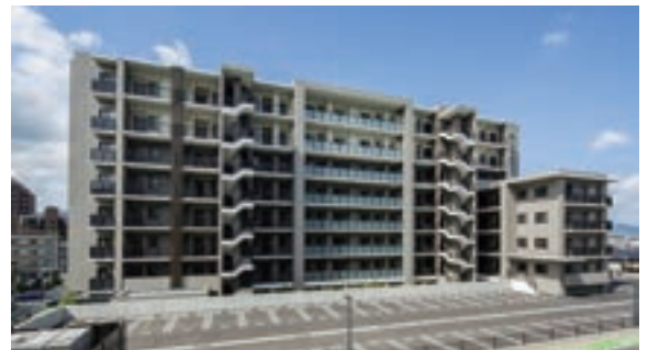
LANDIC HOLDINGS Co., LTD. Tentative name: Nagaoka 2-chome Plan Construction Project (Fukuoka Prefecture)
