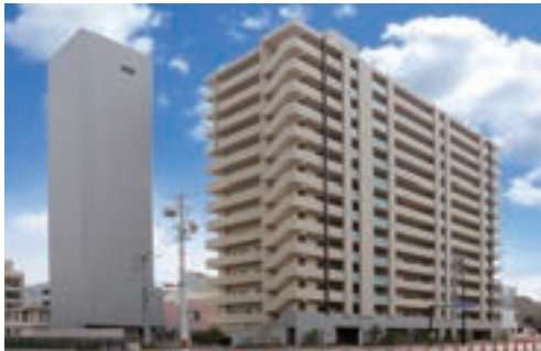
Anabuki Kosan Inc. Tentative name: Alphastates Narukozaka Construction Project (Shizuoka Prefecture)
