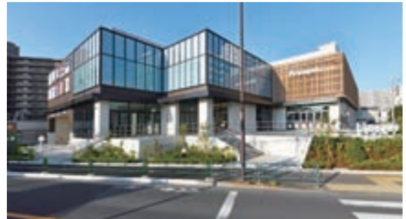
JX Nippon Real Estate Corporation and Daiwa Lease Co., Ltd. Tentative name: Frespo Hibarigaoka Construction Project (Tokyo)
