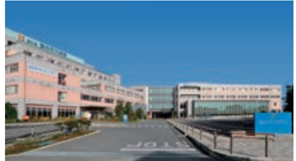
Shijinkai Kenotokorozawa Hospital
