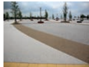
Landscape paving using a natural-color paving mix
