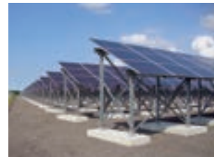
Ballasting at power generation facilities using recycled roadbed materials
